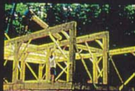
Ken Vilcens of Dover Building smooths a peg in preparation for the raising by crane of the massive bents. Large open spaces with the warm glow of natural wood is one of many "looks" offered by timber frame construction.
