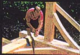
Ken Vilcens of Dover Building smooths a peg in preparation for the raising by crane of the massive bents. Large open spaces with the warm glow of natural wood is one of many "looks" offered by timber frame construction.
